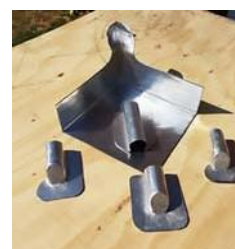
Bossed tinned lead details showing tinned face upwards
